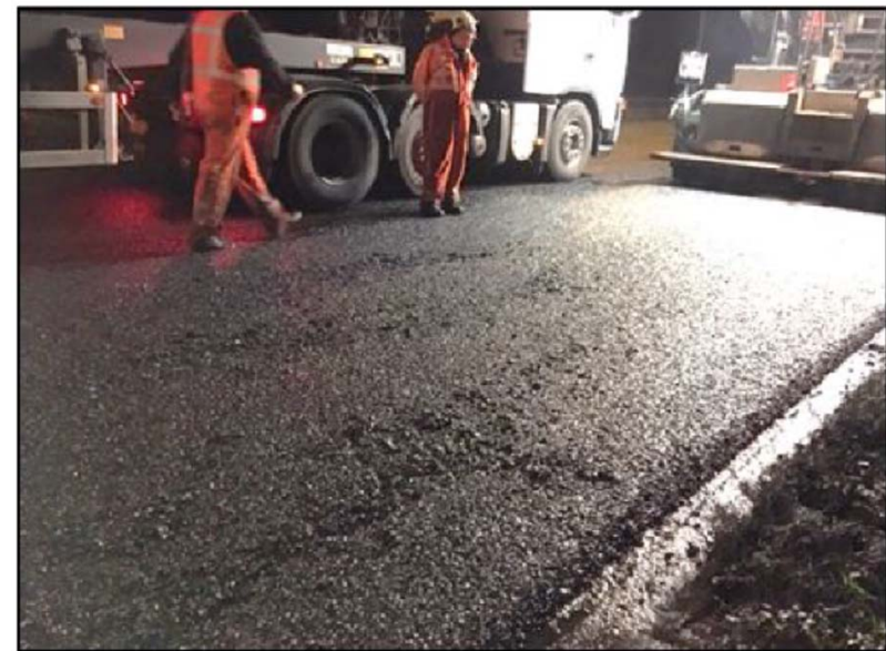
Asphalt with poor adhesion with PmB binder
