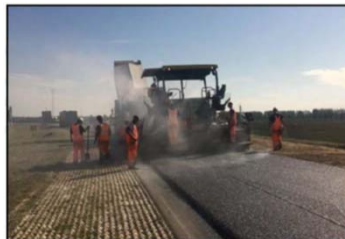
Fume during asphalt laying
