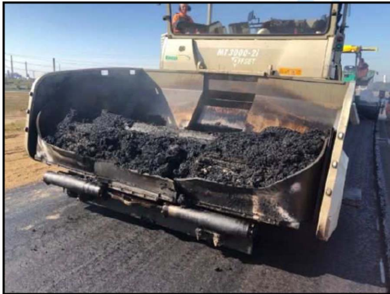
Unworkable asphalt mix with PmB binder
